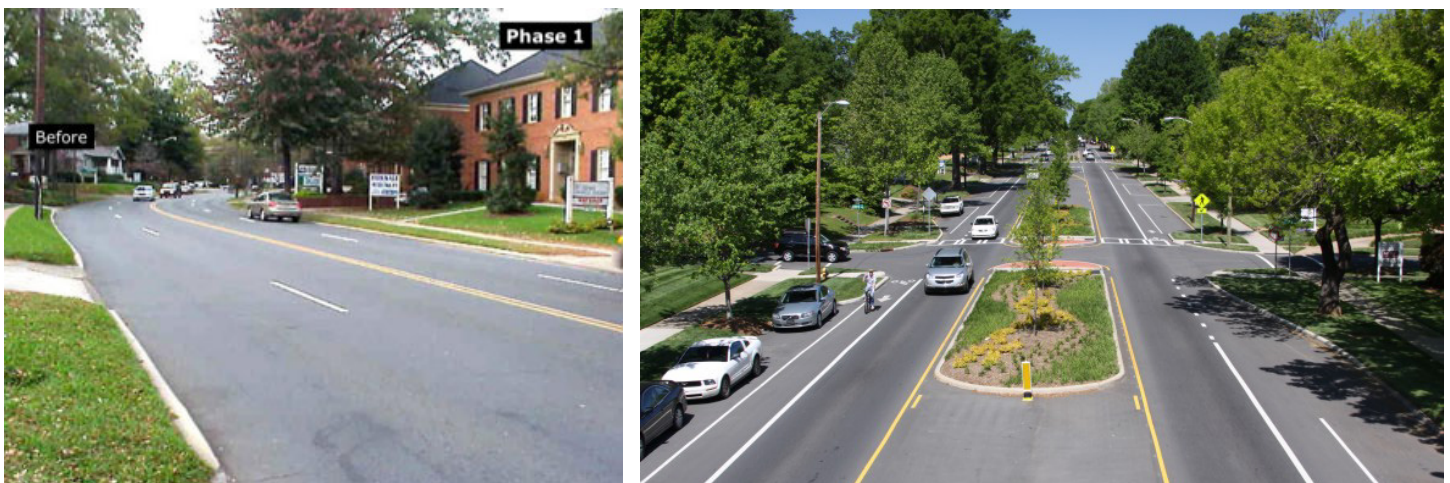
Above: An example of a 4- to 3-lane road diet in Charlotte to make space for bike lanes
