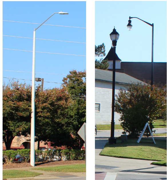
Examples of street and pedestrian lighting. Left, typical Duke Energy smooth fiberglass pole and LED Roadway fixture, to be used town-wide. Right, typical pedestrian and street light for Downtown Village District; pedestrian light is the Mitchell LED Top Hat with ribs, bands, and medallions with 16 ft mounting; post is a Decorative Aluminum Style VI; street light is a Teardrop LED on a Decorative Tapered Metal pole in black.
