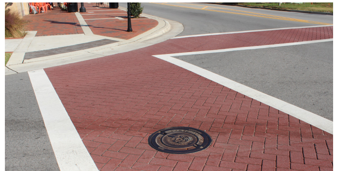
Crosswalks: Typical stamped and surface coat treatment asphalt. Surface color applied with Endurablend or equal product. For use town-wide and Downtown Village District
